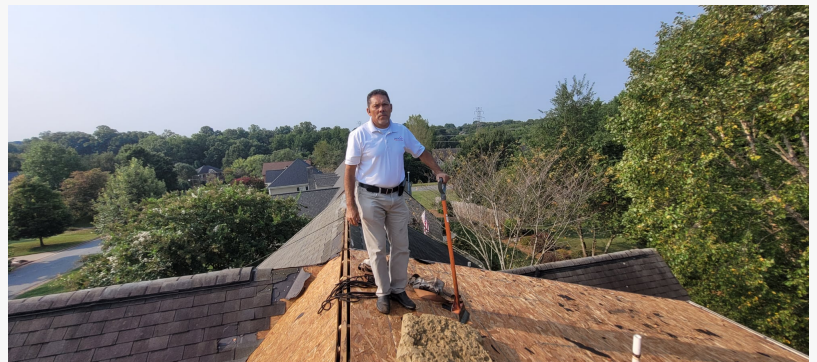
Southland Roofing Roofing Installation
