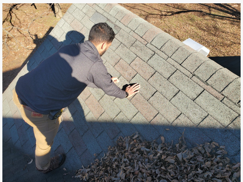
Southland Roofing Roofing Repair
