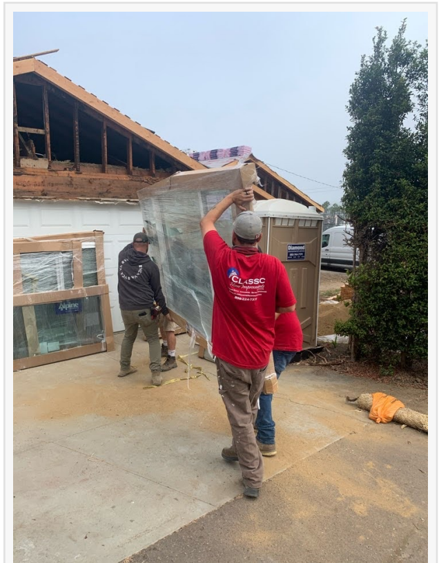
Laborers Working on a Remodeling Jobsite
