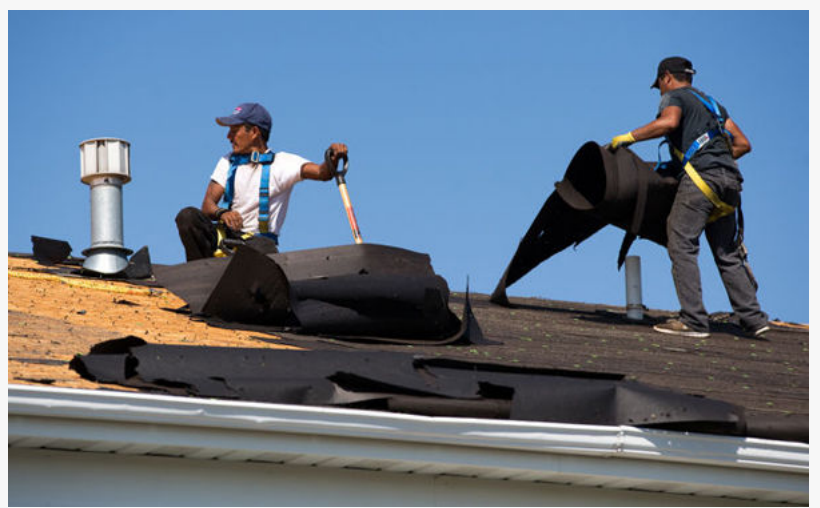
Latino construction workers rebuilding a roof
