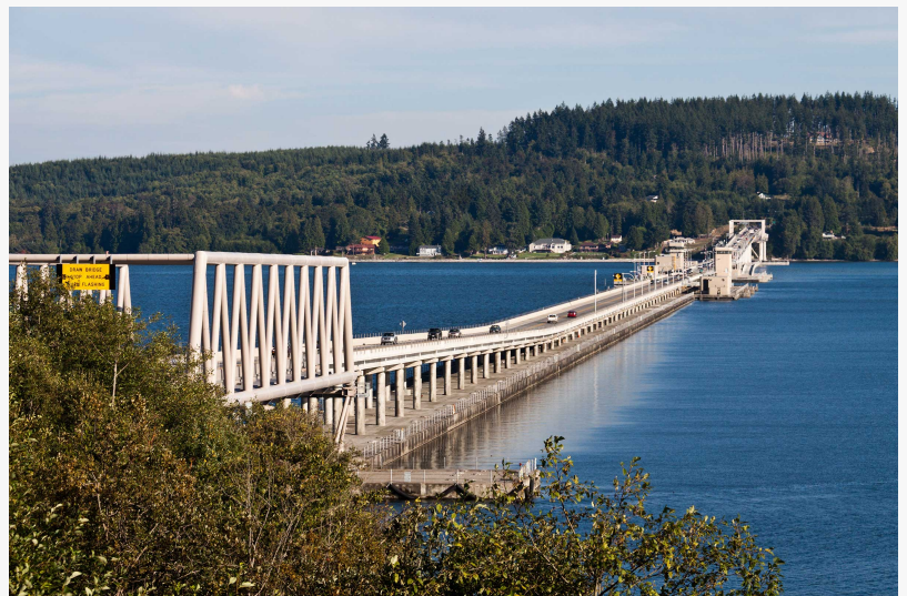
Hood Canal Bridge
