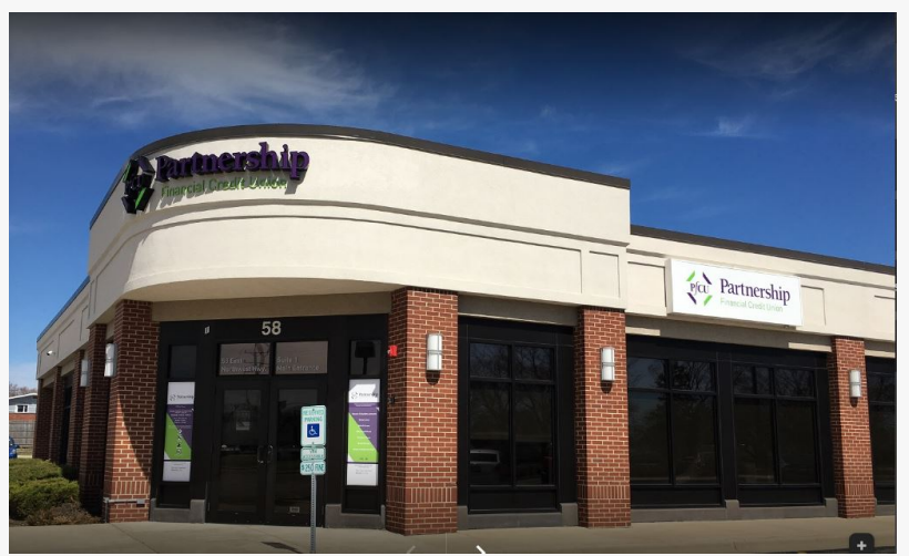
PFCU location in Des Plaines, IL
