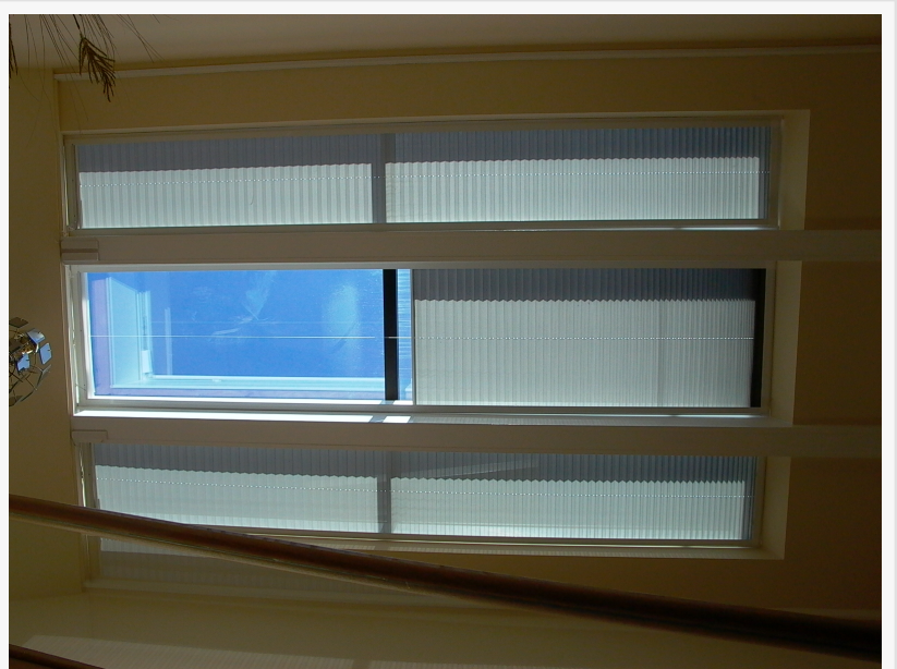
Skylight motorized shade
