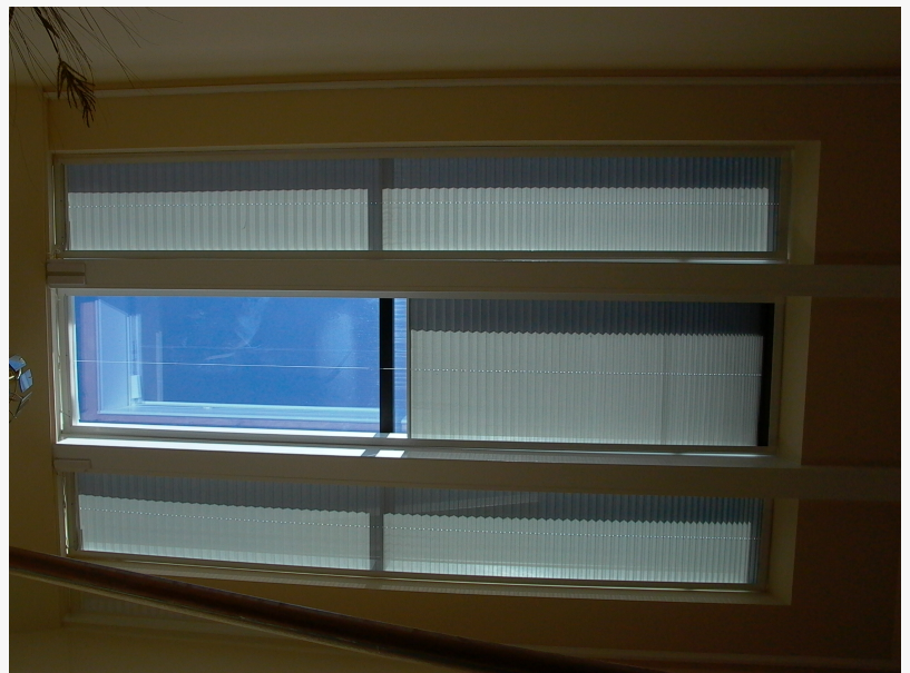
Motorized skylight screens
