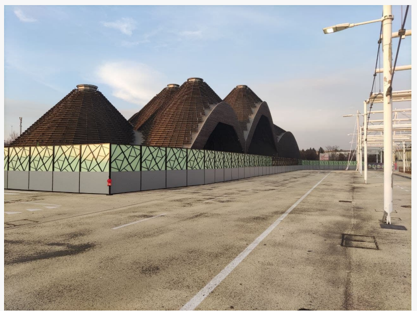
Sound absorbing panels at MIND in Milan
