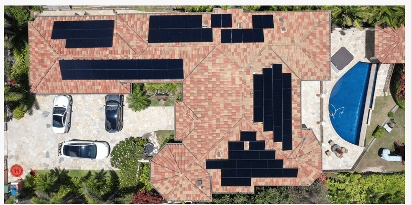
Sunspare Residential Installation
