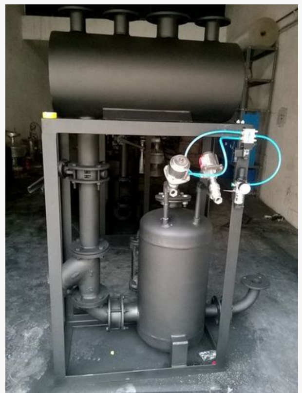
Condensate Return Pumps Market Size, Trends And Forecast To 2031
