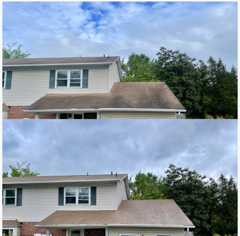
All Clean Power Wash LLC Roof Cleaning
