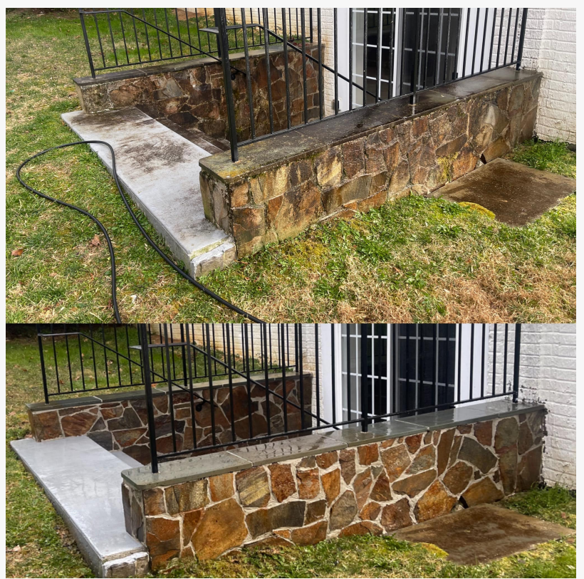
All Clean Power Wash LLC Surface Cleaning
