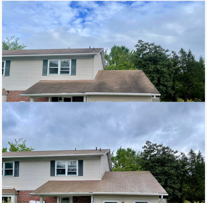
All Clean Power Wash LLC Roof Cleaning
