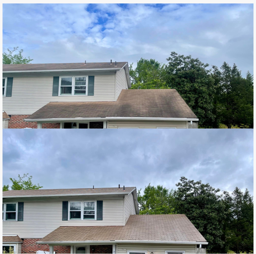
All Clean Power Wash LLC Roof Cleaning
