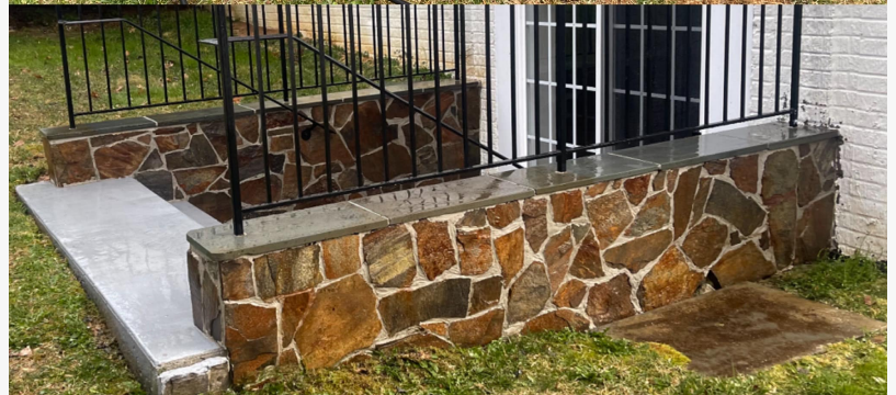
All Clean Power Wash LLC Surface Cleaning
