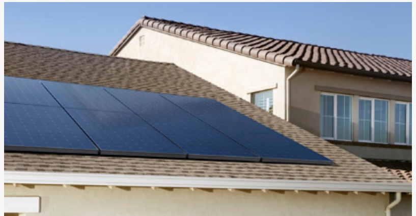
Better Solar Solution Rooftop Solar
