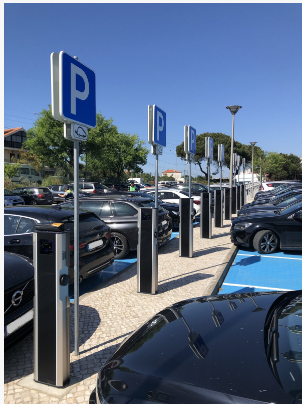
CityCharge V2 installed in Portugal
