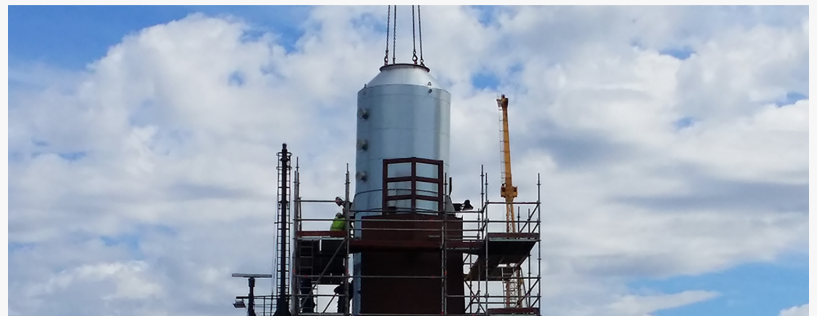
Retrofitting Scrubber into Vessel
