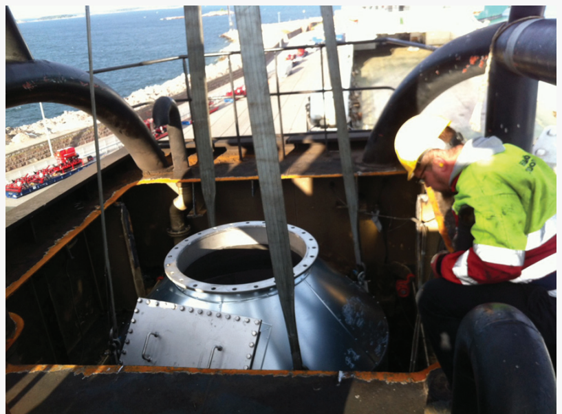
Scrubber Retrofitting Process
