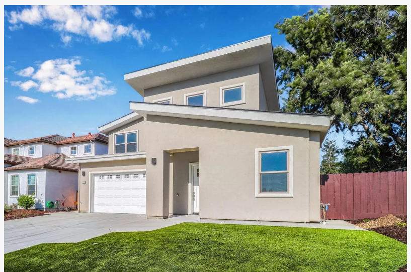
SIDCO's fire-resistant home in Hollister, CA
