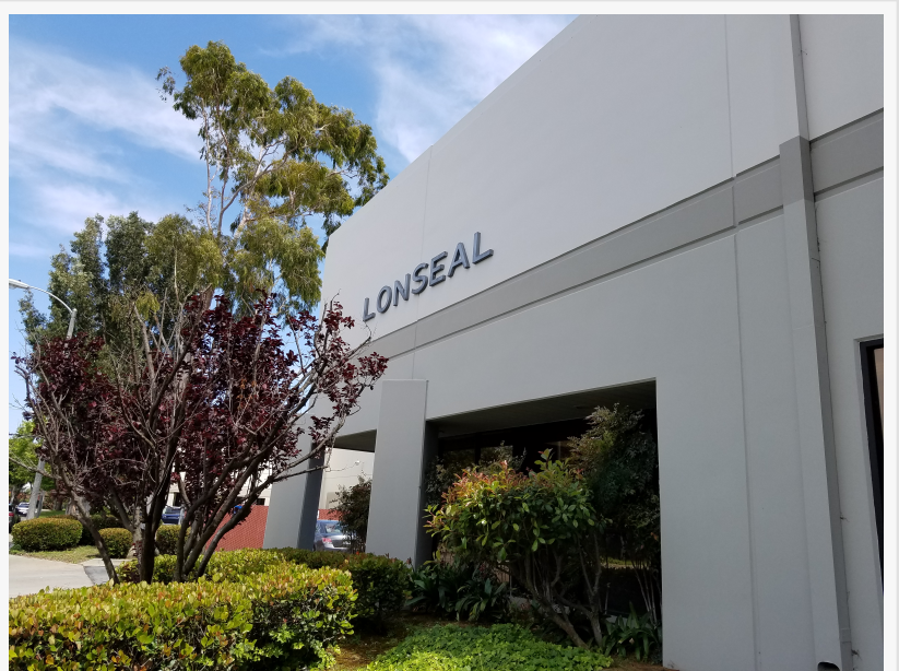
Lonseal Office in Carson, CA
