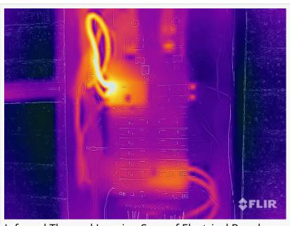
Infrared Thermal Imaging Scan of Electrical Panel
