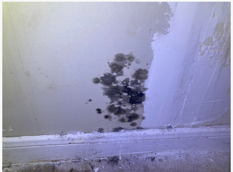
Hidden Mold Growth Behind Wall
