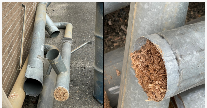
Woodshop Dust Collector Maintenance Required
