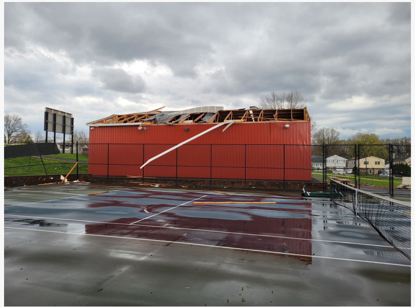
Bergenfield NJ - roof of storage building destroyed by microburst
