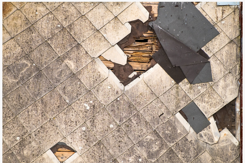
A mixture of asbestos and cement was used to produce roof shingles for decades throughout the twentieth century.
