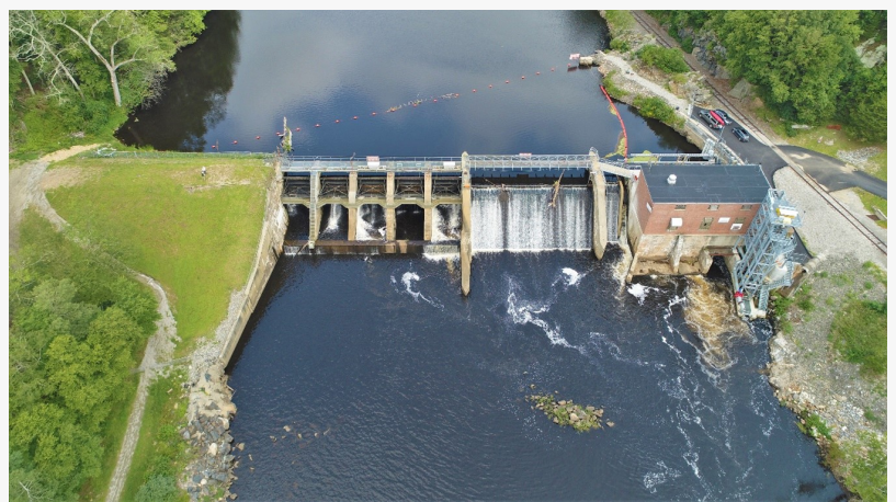
Scotland Dam Generating Station
