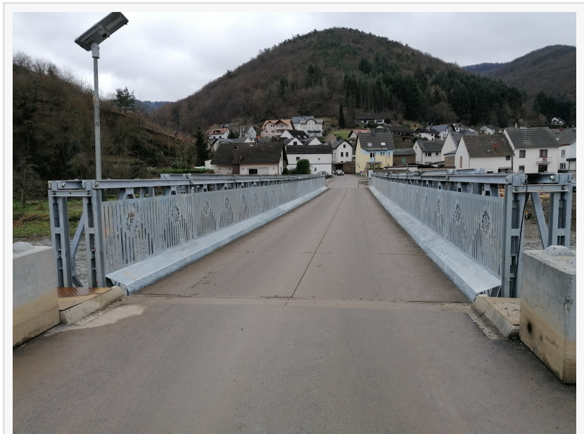
Mabey Bridge in Germany - Image courtesy of THW
