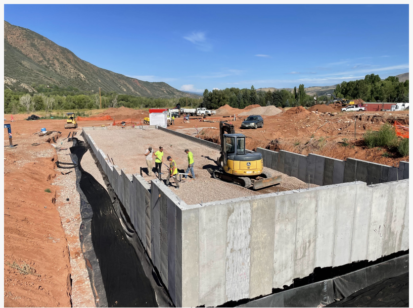
Construction progresses on Aspen Distillers' distillery.
