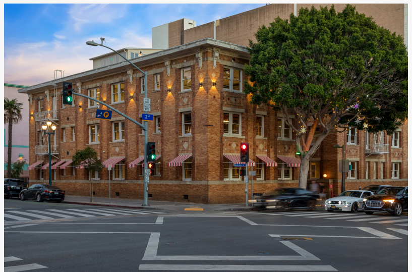
1305 2nd Street after completion of a full building restoration
