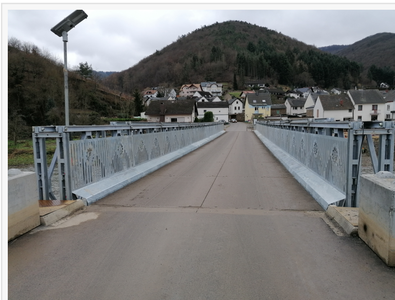
Mabey Bridge in Germany - Image courtesy of THW
