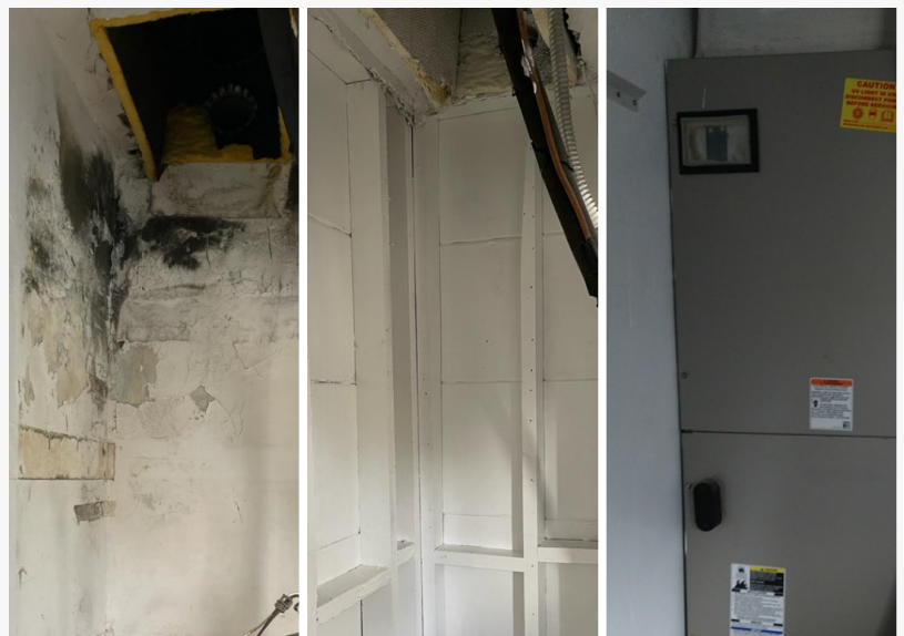
AC Closet Before and After Mold Removal
