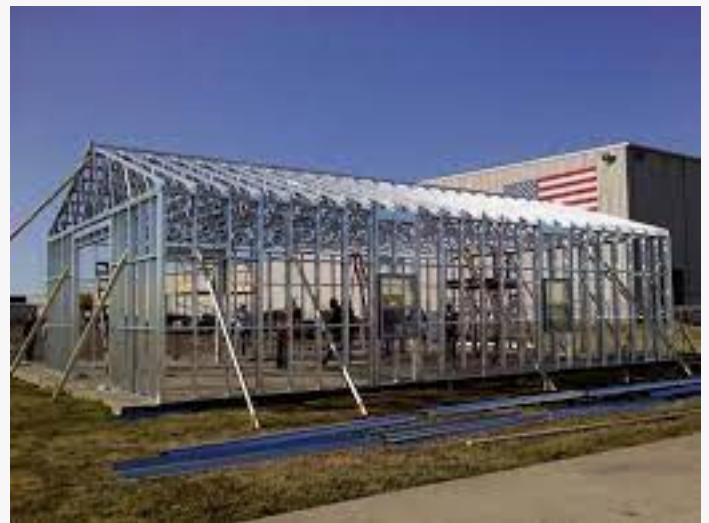
Pre-engineered Building Market Demonstrates A Spectacular Growth By 2031
