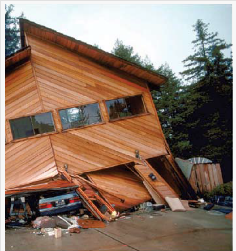
foundation repair in LA
