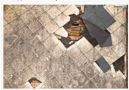
A mixture of asbestos and cement was used to produce roof shingles for decades throughout the twentieth century.
