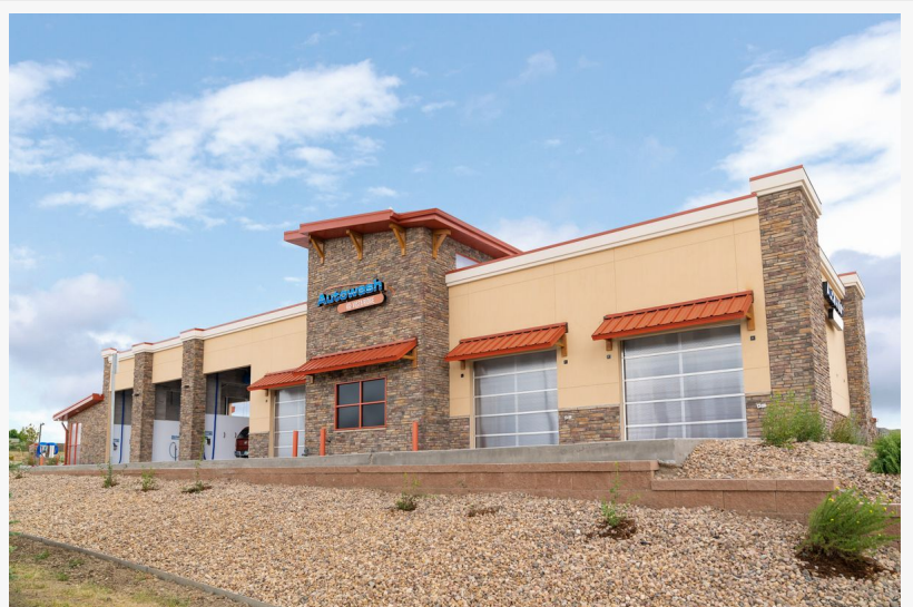
The new Autowash located at 530 Commons Drive in Erie, CO.
