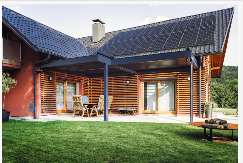
Energy Plus Solar Installation
