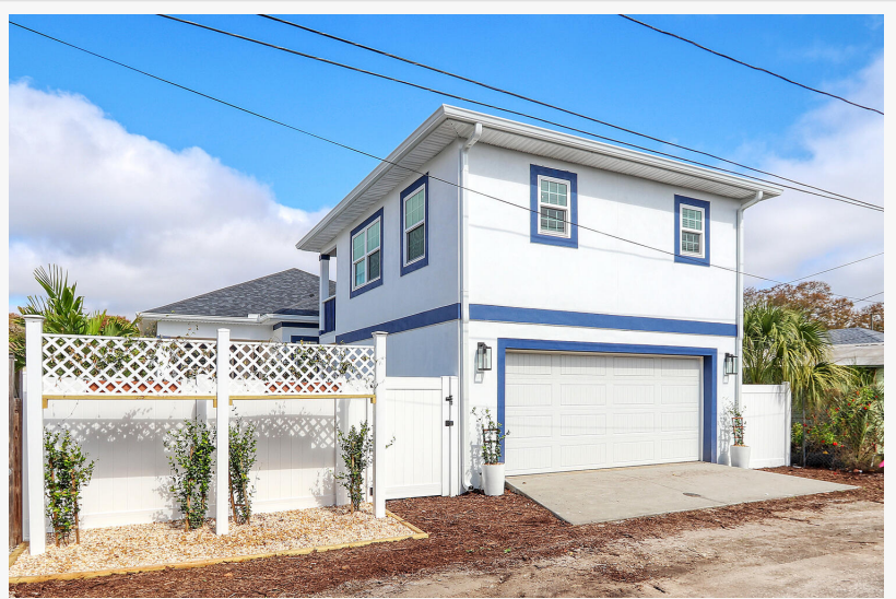
Already completed St. Petersburg Carriage Home with 2-car garage
