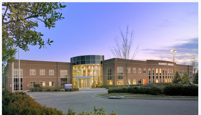
The Market America Headquarters in North Carolina
