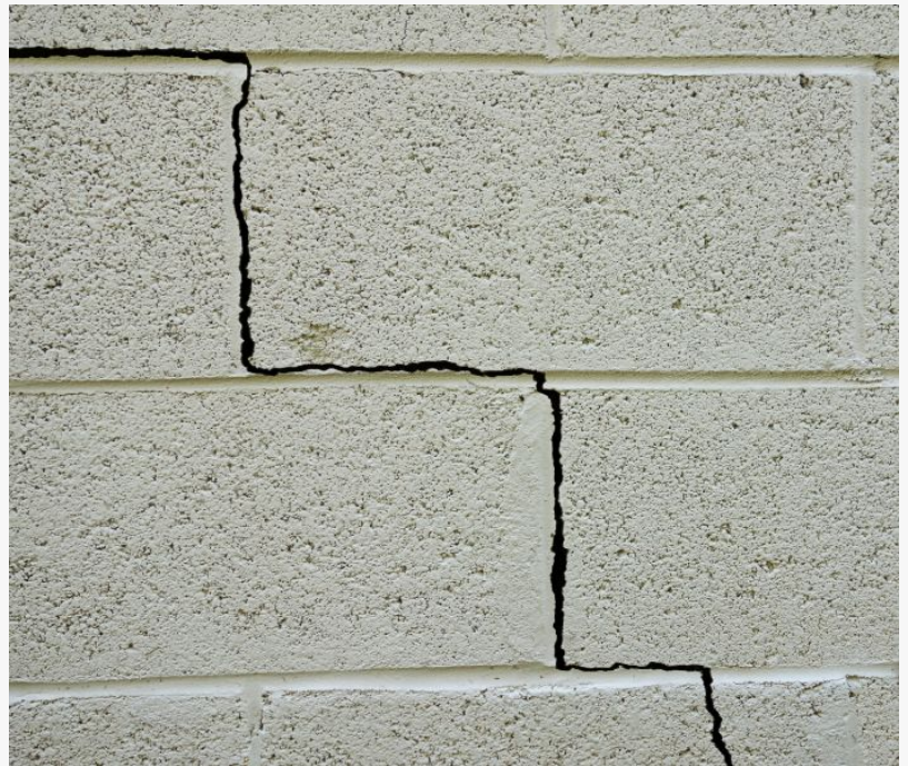
Peoria home requiring a stair-step crack repair
