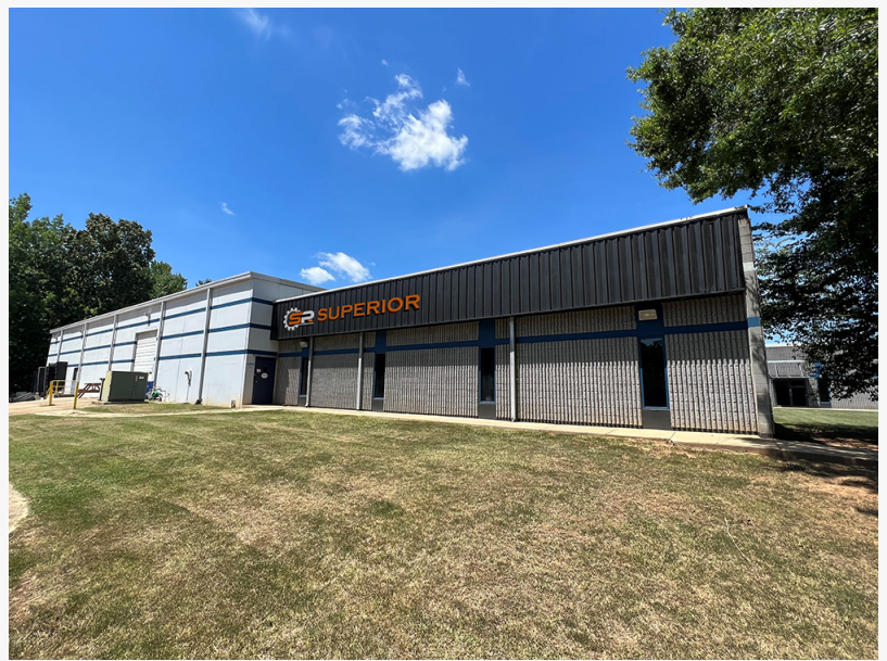
SPR's New East Coast Distribution and Rental Facility
