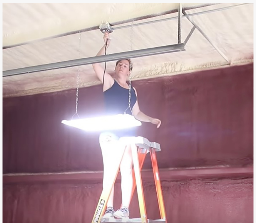
April Wilkerson installing a PLT Solutions LED High Bay
