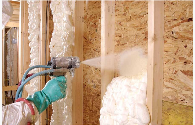
Spray Foam Insulation Process
