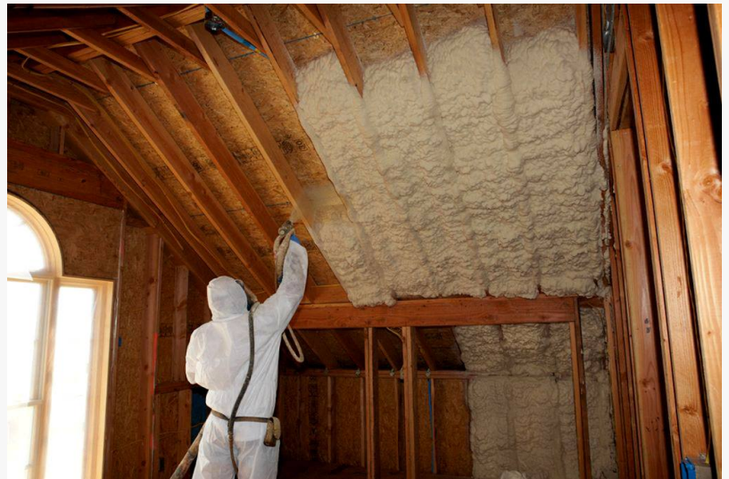
Professional Spray Foam Insulation Services
