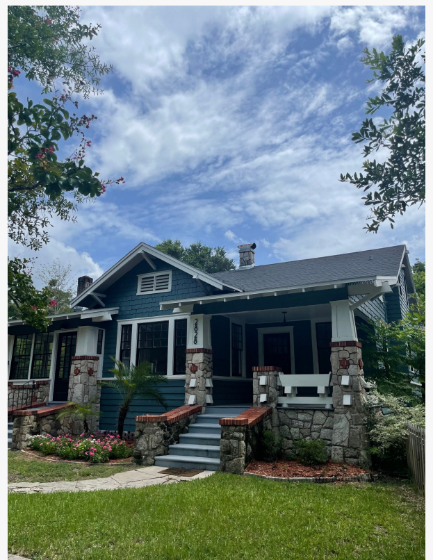
EASTERN ROOFING COMPANY ROOFING PROJECT
