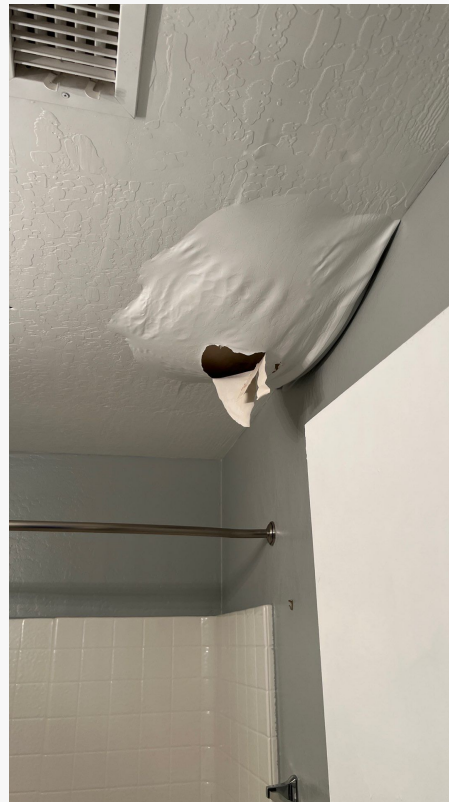
This A/C Leak caused a large bubble in the ceiling drywall.
