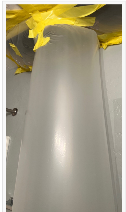
Technician cut out the damaged drywall and set up a containment tube to direct airflow for dry out.
