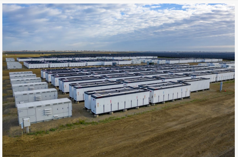
Grid Energy Storage Market Size 2022
