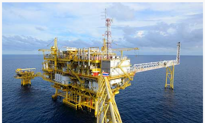
Drilling Chemicals Market Analysis
