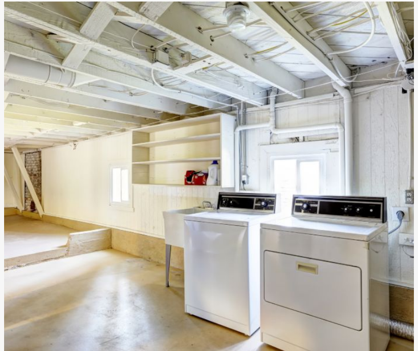
Home after the basement is waterproofed
