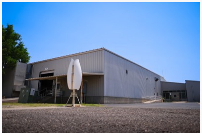
Flower Turbines Outside Manufacturing plant
