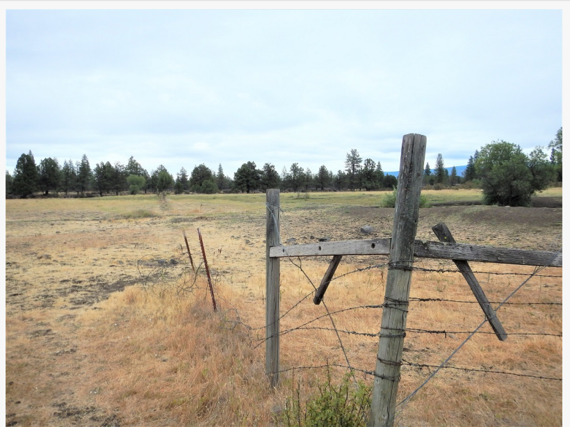
Example of one section of the OR-CA state line fencing that is down
