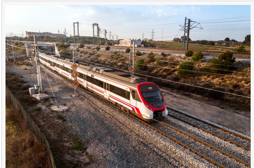
The Automatic Train Control Market
