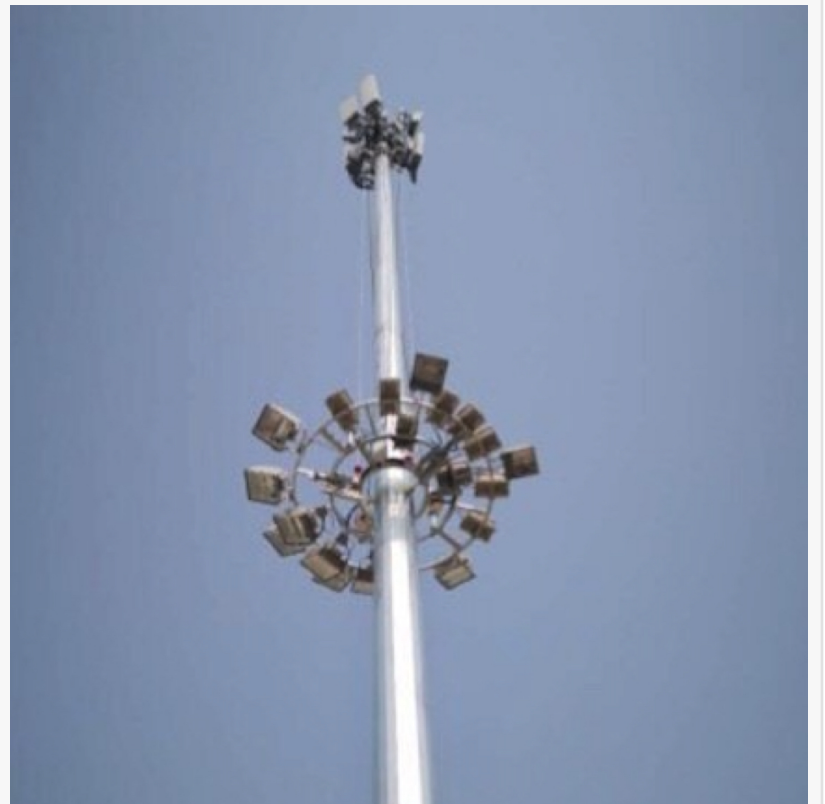
High Mast Light Pole with Raise-Lower Rack System
