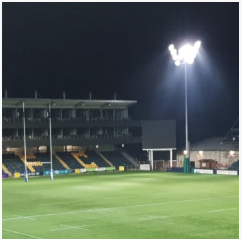
High Mast Light Poles at a Small Stadium
